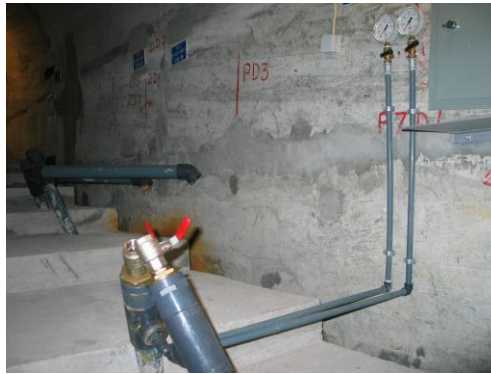
Figure 66: Piezometer in the foundation
